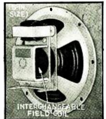
Interchangeable-field speaker. (1191)
